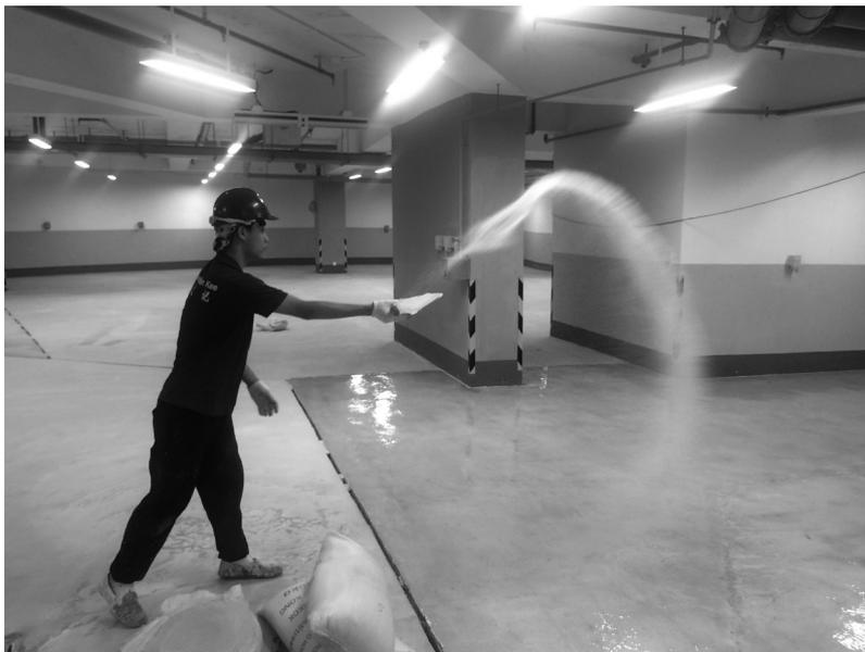
(vii) Removing excess quartz sand from the primer
