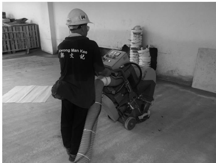
(iii) Surface preparation – repairing surface cracks
