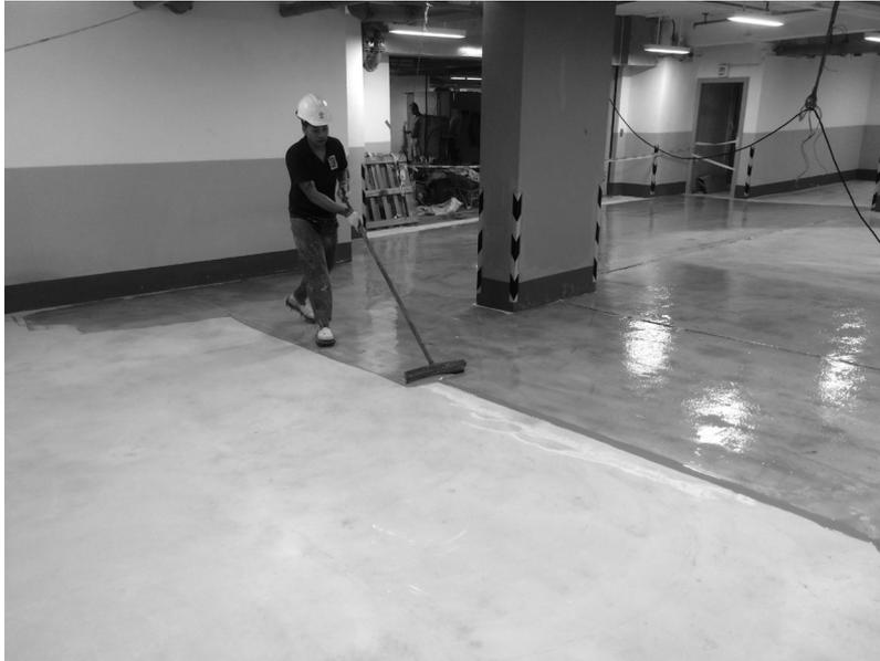
(vi) Sprinkling quartz sand onto the primer to create friction
